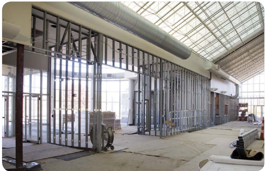
Construction continues on the new North Royalton Family YMCA.
