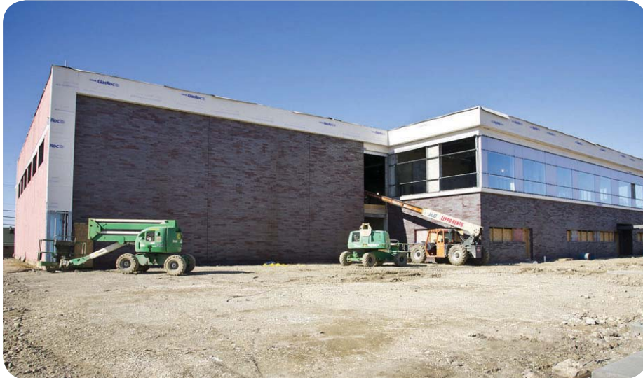
The new Warrensville Heights Family YMCA under construction.
